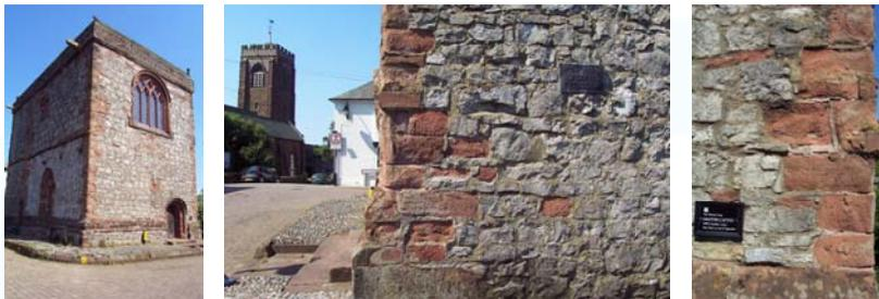
The National Trust chose an NHL 2 to provide certain durability to the moderately exposed conditions but provide maximum breathability. Samples of mortar analysed by the Scottish Lime Centre showed a mixture of non-hydraulic to eminently hydraulic, but the Trust felt a NHL 2 was a suitable compromise to give adequate strength with the best possible breathability.
